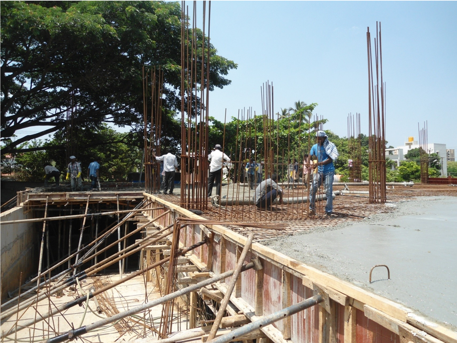
RCC roof casting for the basement slab in progress, 14.4.2019
