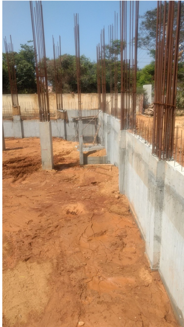
Retaining wall of the basement, 13.2.2019
