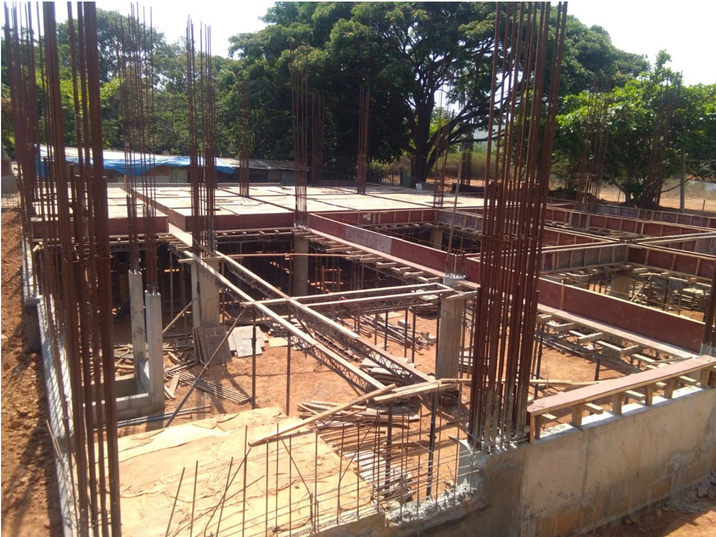
Preparatory work for the casting of the RCC roof slab for the basement , 12.3.2019
